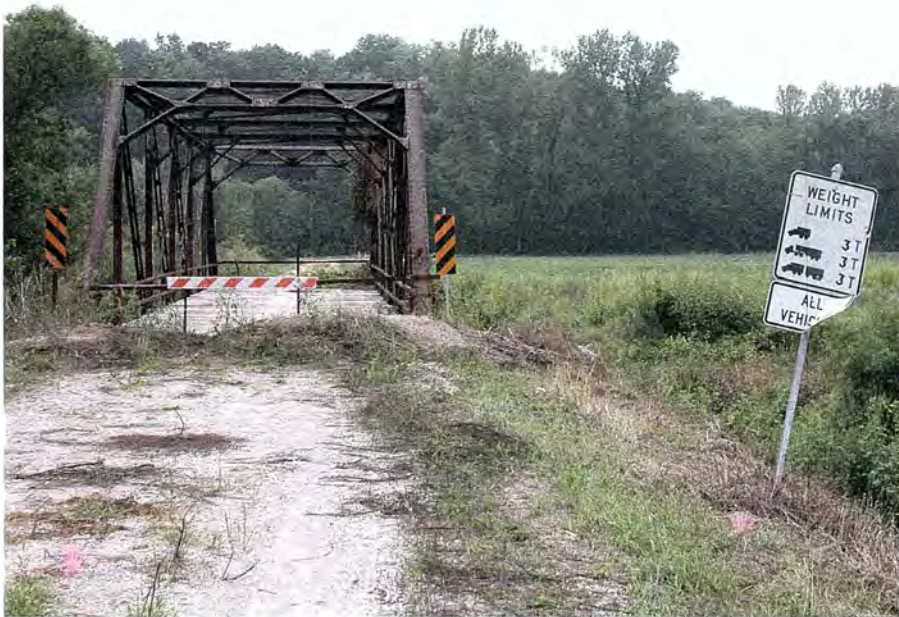
Figure 1.1. Wapello County truss bridge prior to replacement.
